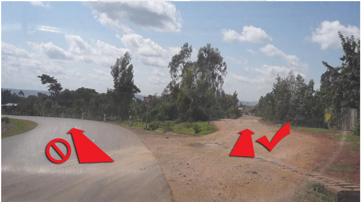
Picture: Showing the -T-type road at Megara; the arrow shows as there gorge that vehicles are rollover as driver thinks the way is street.
